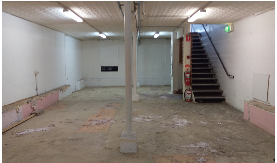
Hellbound, before renovation
